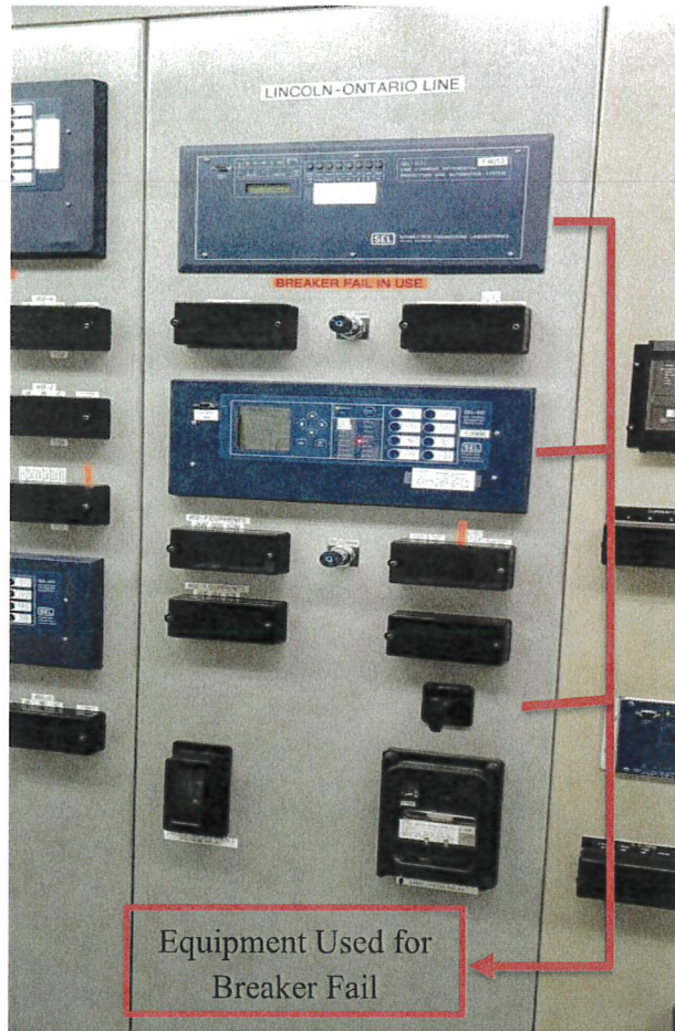
4527 Breaker Fail Addition @ Lincoln Substation
