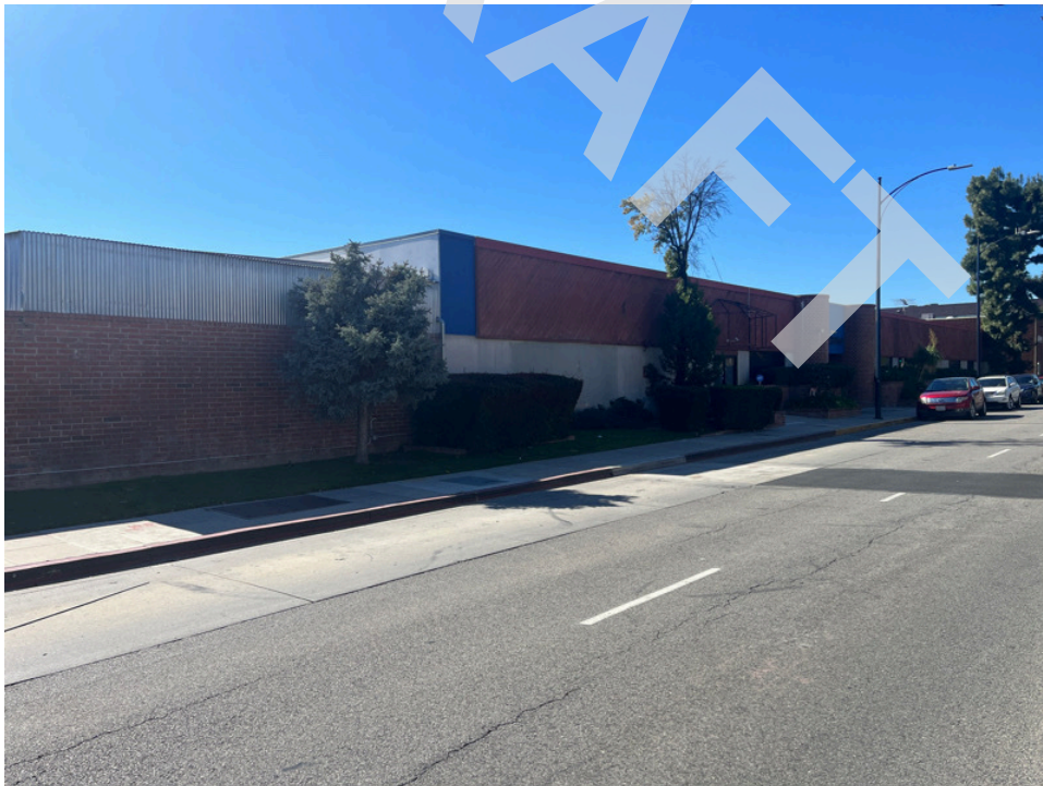
14. South-adjoining property (3000 West Empire Avenue)
