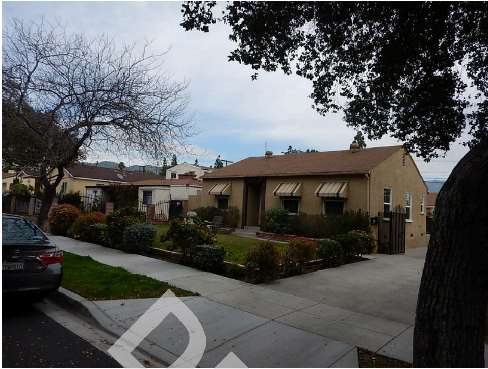
15. View of adjacent site on northeast side of subject property
