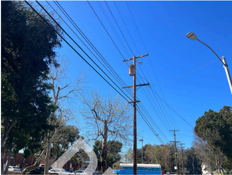
9. Pole-mounted transformer
