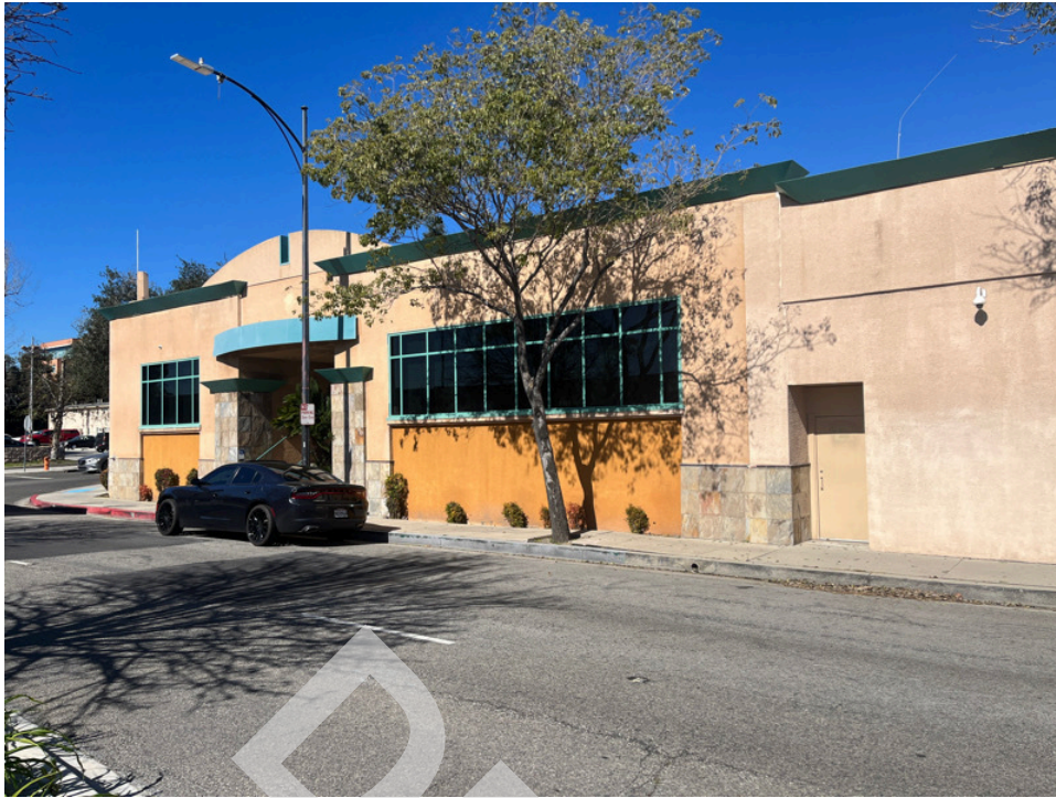
13. East-adjoining property (2919 West Empire Avenue)
