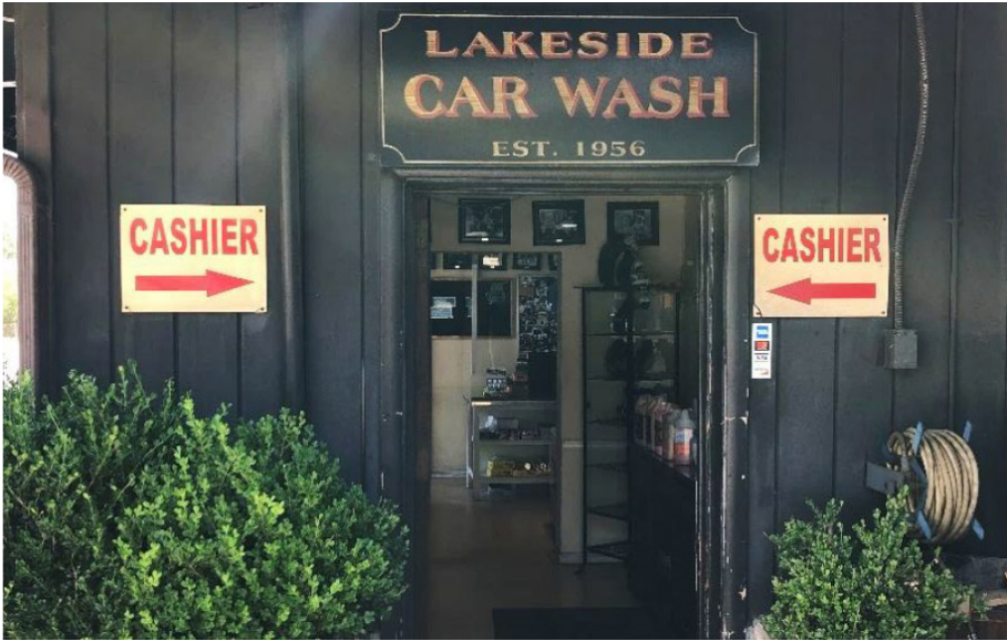
View of the main bay west elevation, facing east.
