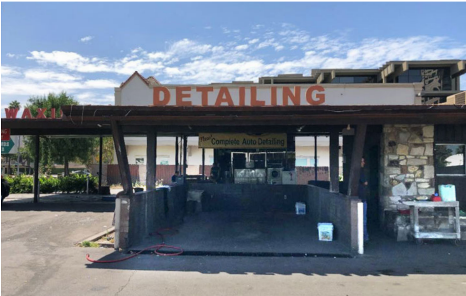
View of the detailing bay, facing south.
