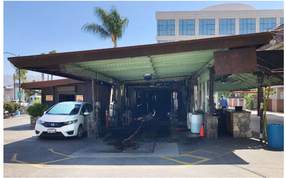
View of the main bay and car wash west elevation, facing east.
