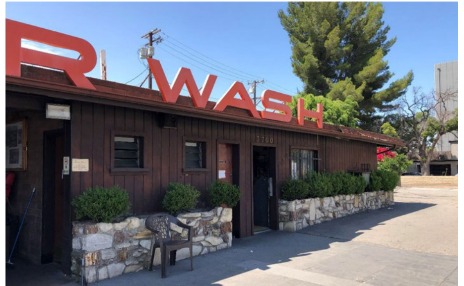
View of the main bay, facing southwest.
