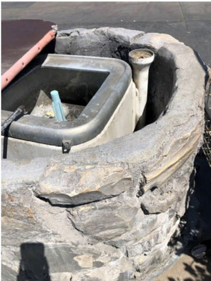
Detailed view of the rock planter/gas pump, facing northwest.
