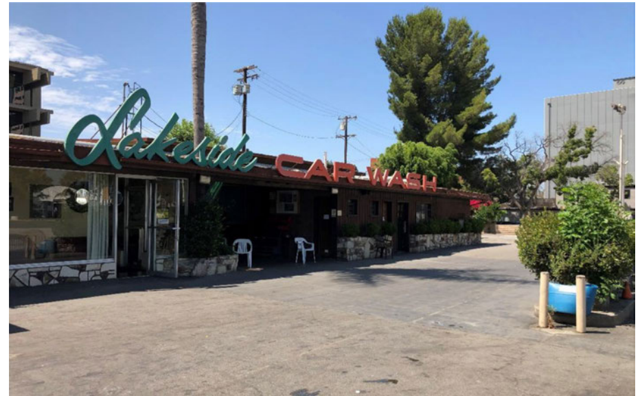
View of the main bay, facing southwest.
