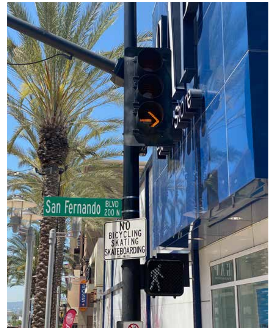
Flashing Right-Turn Arrow and Advance Walk on San Fernando Blvd. and Palm Ave.
