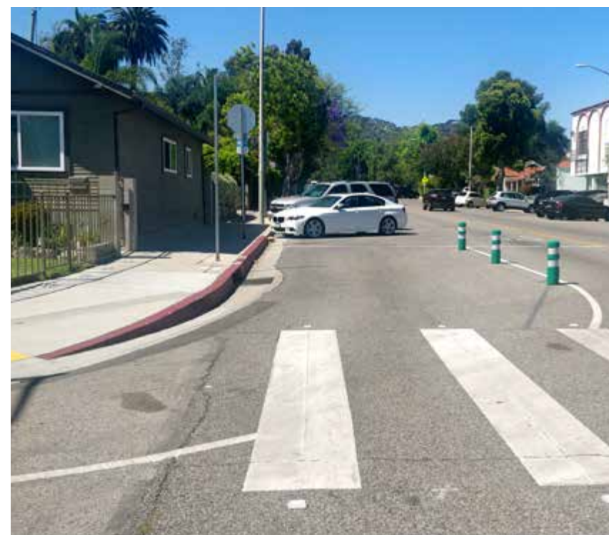
Demonstration/Interim Installation of a Curb Extension.
