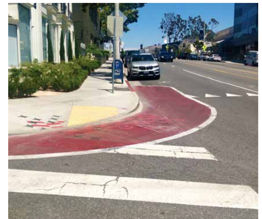
Demonstration/Interim Installation of a Curb Extension.
