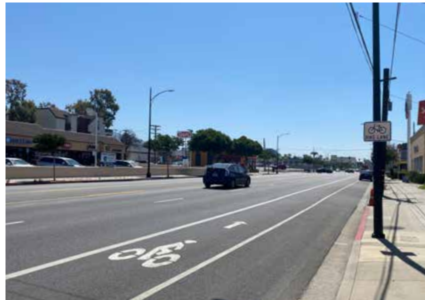
Class II Bikeway (Bicycle Lane) on San Fernando Blvd. near Bethany Rd.
