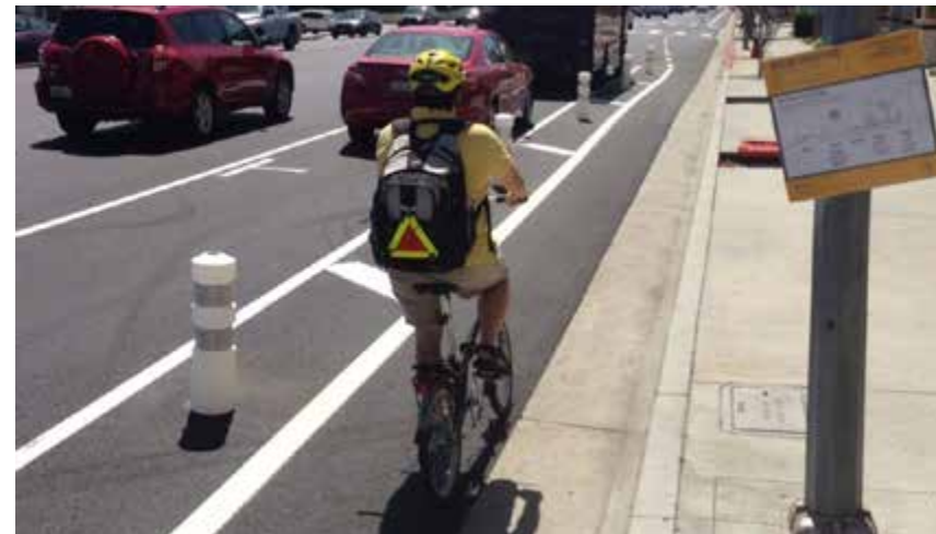
One-Way, In-Street Class IV Bikeway, Adjacent to On-Street Parking, Protected by Bollards and On-Street Parking (Source: laststreetsblog.com).
