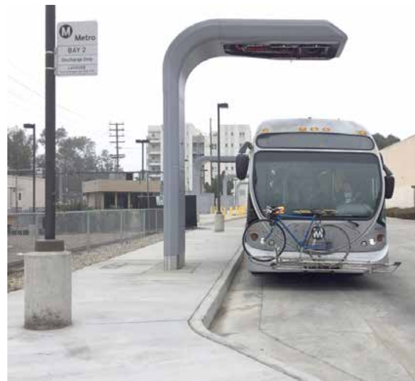
Electric Bus Charging Station (Source: metro.net).
