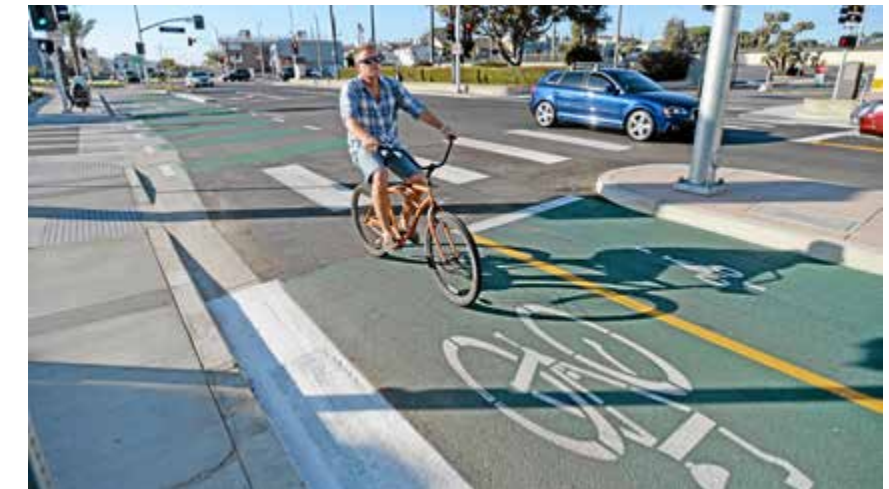
Two-Way, In-Street, Class IV Bikeway (Source: dailybreeze.com).
