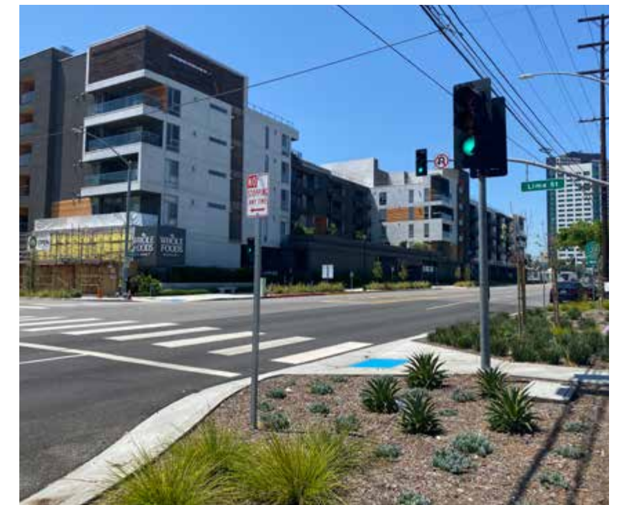
Curb Extension with Landscaping on Alameda Ave. at Lima St.
