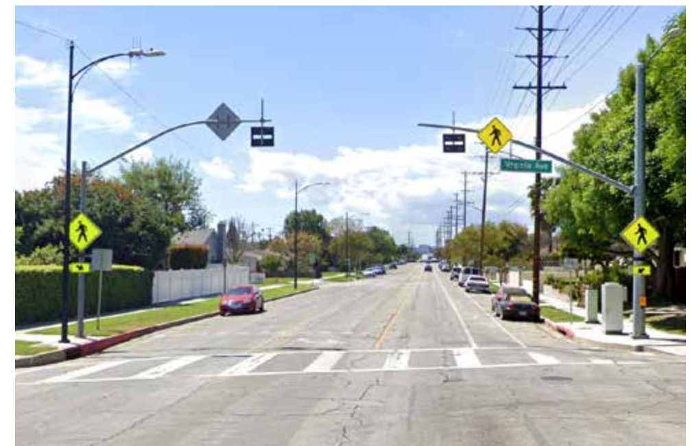
Flashing Beacons with High-Visibility Crosswalks at Virginia Ave. and Verdugo Ave.
