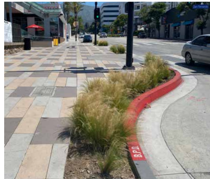
Curb Extension with Bioswale on Magnolia Blvd. at San Fernando Blvd.
