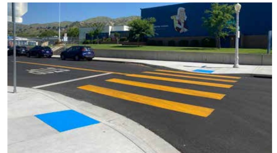
Curb Ramps, Curb Extension, and High-Visibility Crosswalks at 6th St. and Cambridge Dr.
