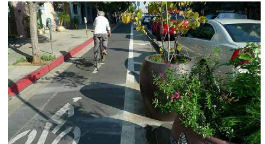
One-Way, In-Street Class IV Bikeway, Adjacent to On-Street Parking, Protected by Planter Boxes (Source: laweekly.com).
