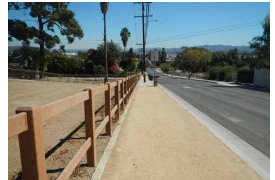
Bridle Path in lieu of a Sidewalk without Side Barrier in Avocado Heights, CA (Source: lacounty.org).
