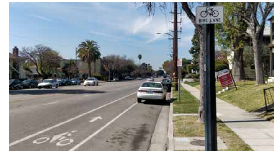
Class II Bikeway (Bicycle Lane) on Victory Blvd. near Catalina St.
