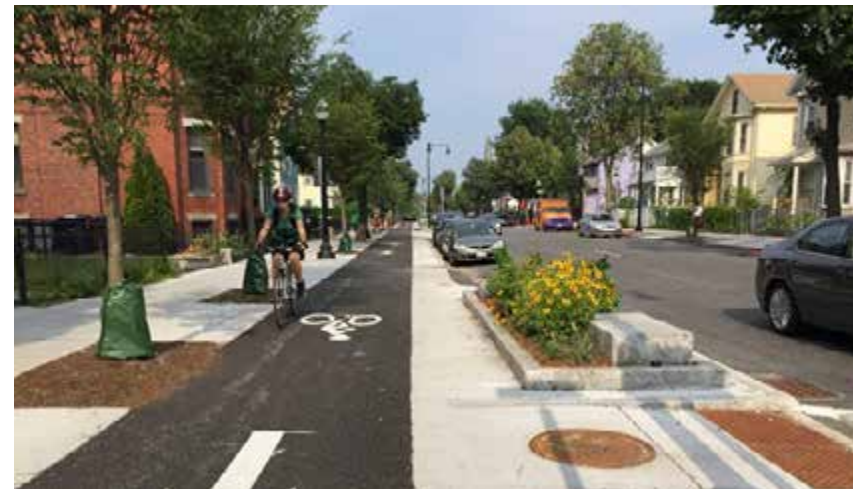
One-Way, Sidewalk-Level, Class IV Bikeway (Source: cambridgema.gov).
