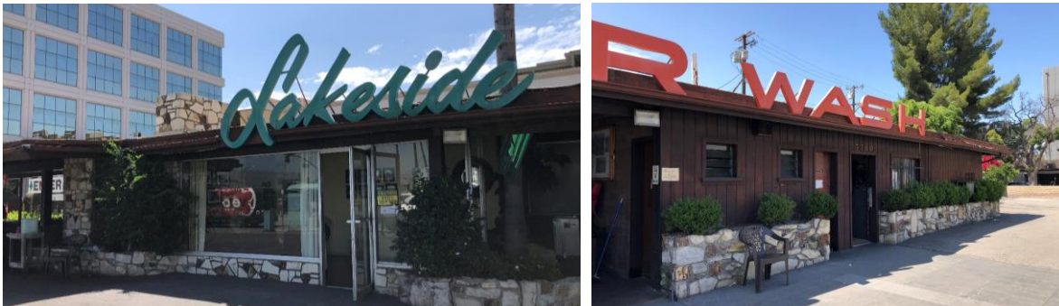
North elevation details, July 2020.
