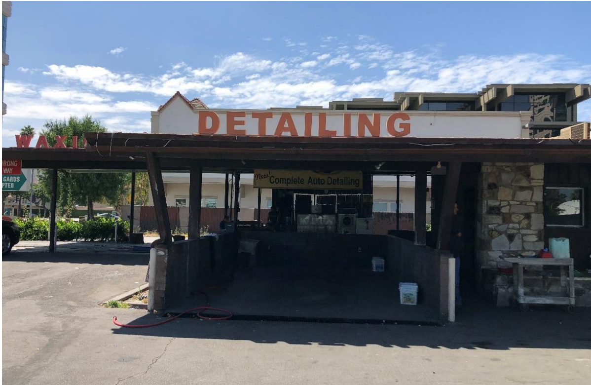
Figure 5 Detailing Bay, Facing South
