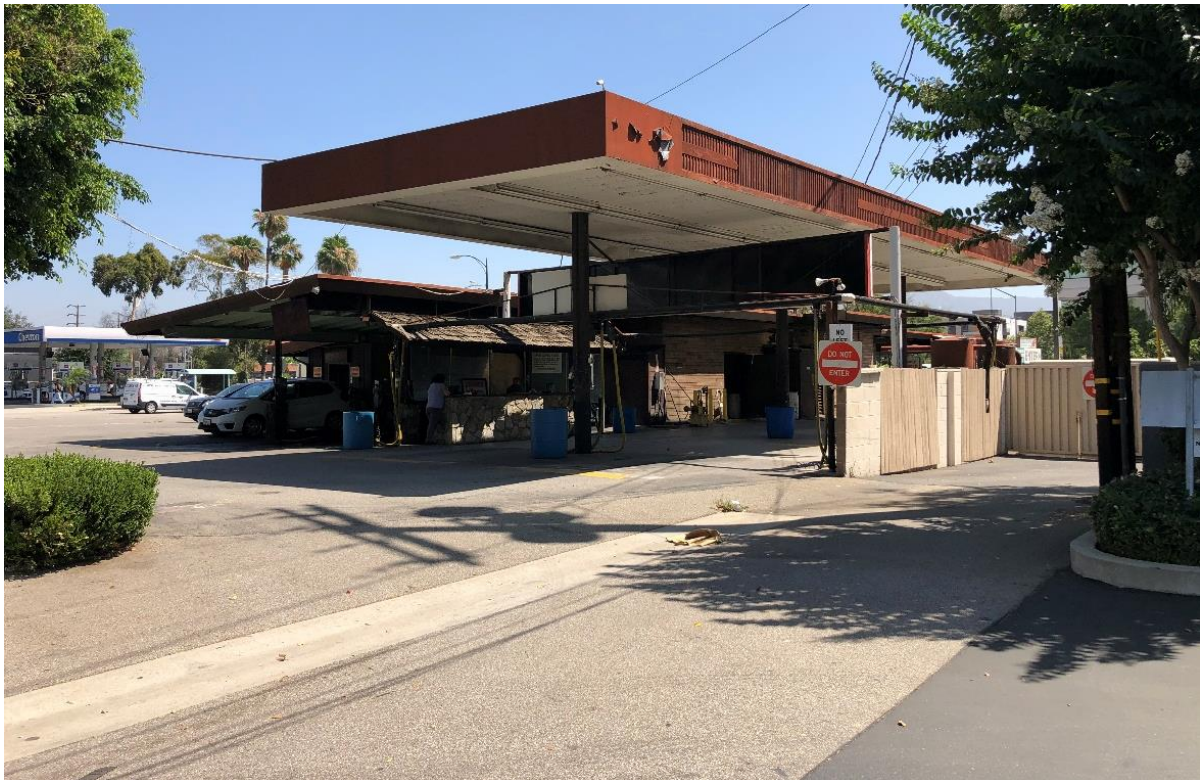
Figure 14 Utilitarian Structure, Facing Northeast
