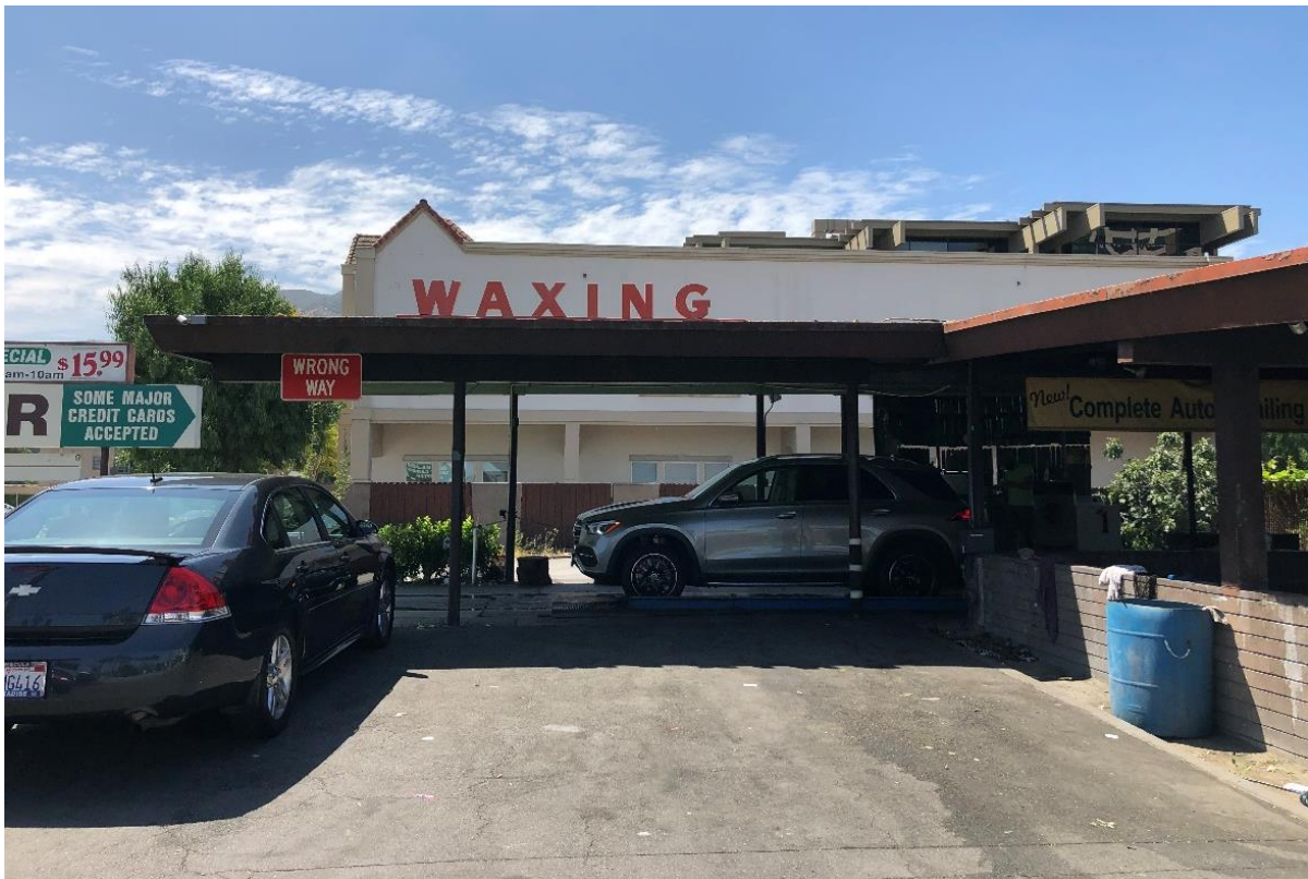
Figure 4 Waxing Bay, Facing South
