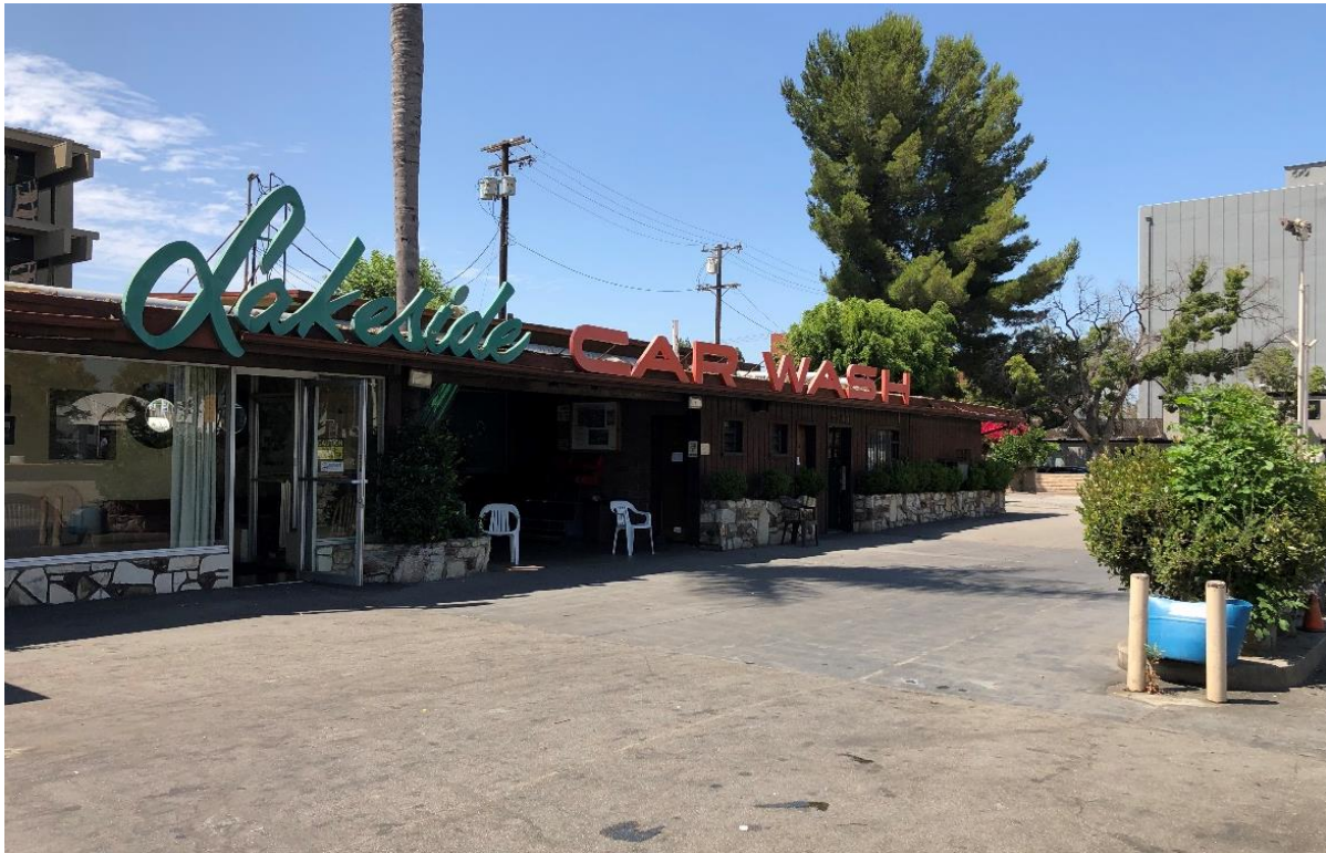
Figure 6 Main Bay, Facing Southwest
