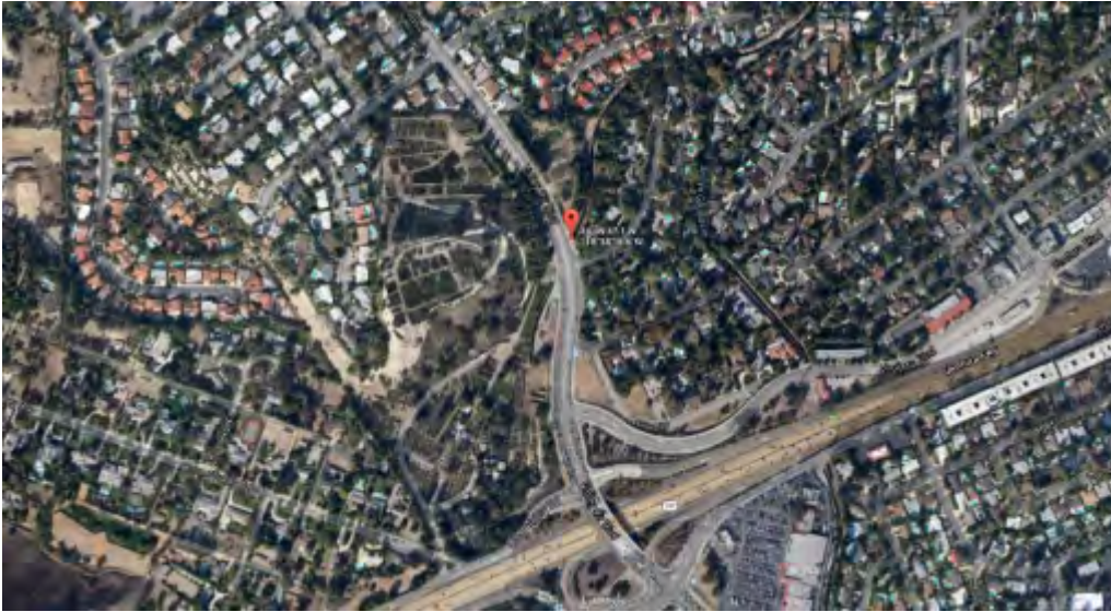
MCC_VAL Aerial View
