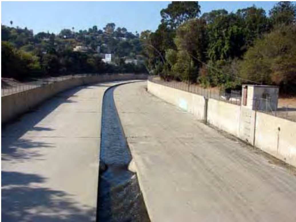
LAR_04_TUJ Ground-Level View
