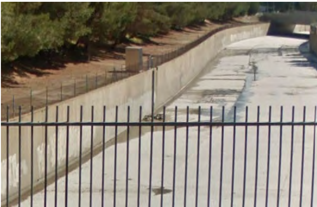
TW_MOO Ground-Level View
