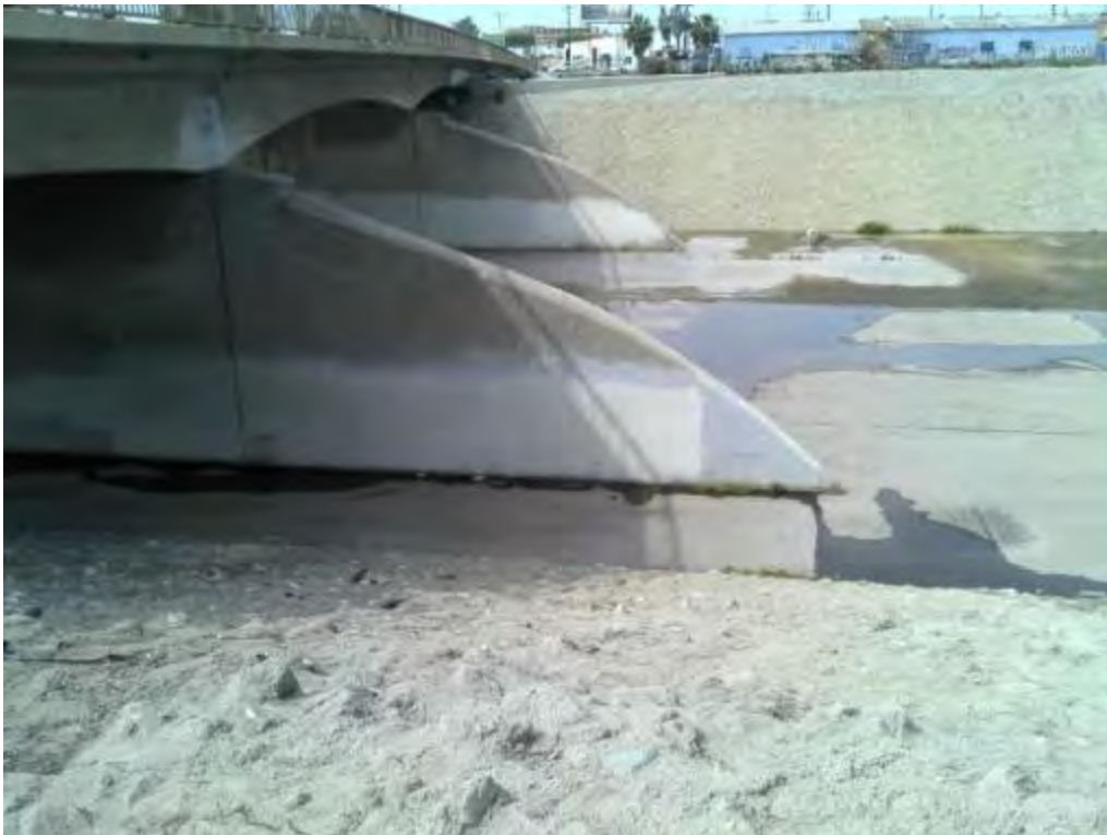
RH_SLA Ground-Level View
