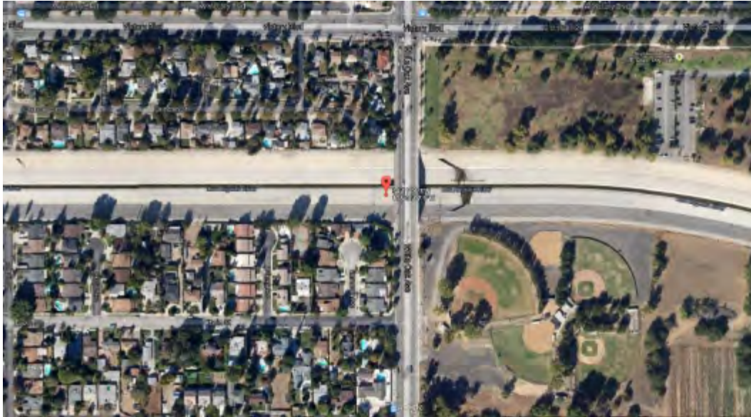
LAR_06_WHI Aerial View
