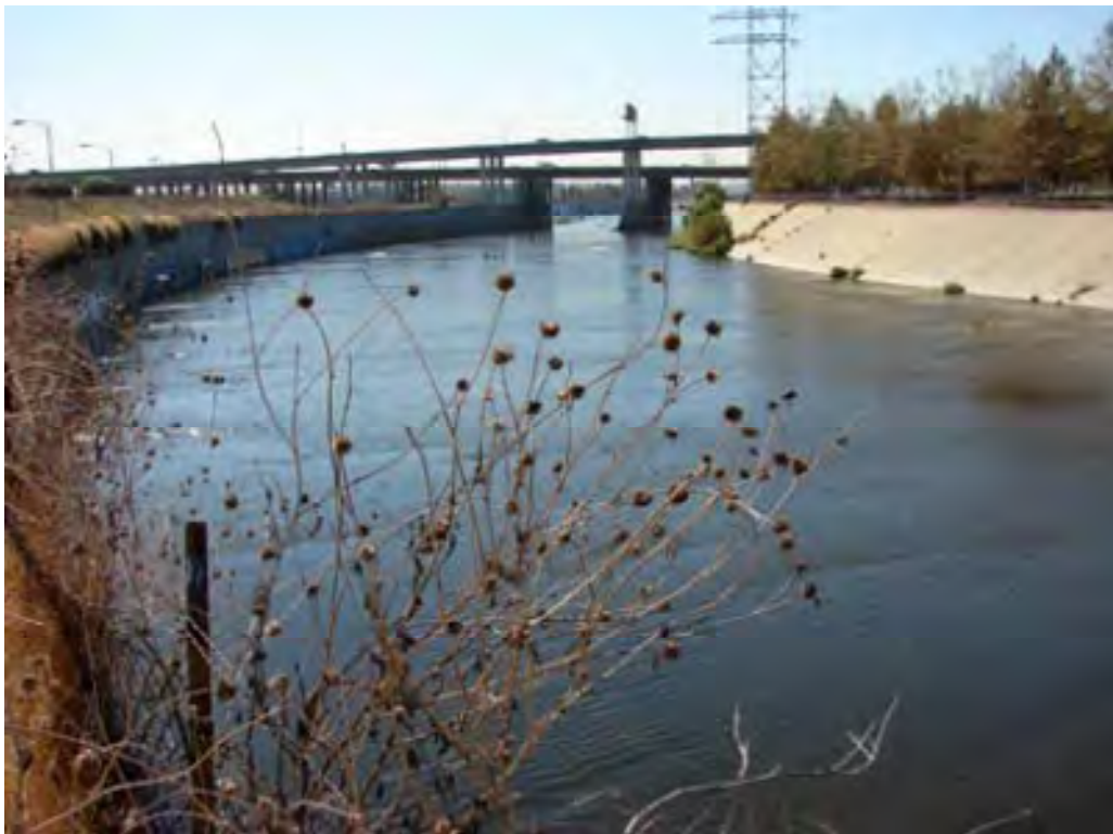
LAR_03_ZOO Ground-Level View
