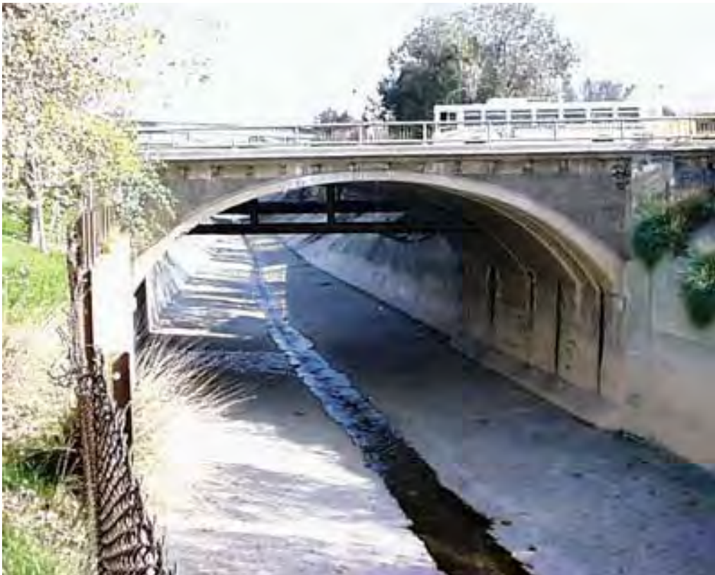
AS_SAN Ground-Level View
