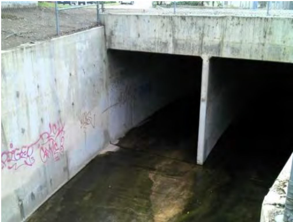
DCC_VEN Ground-Level View
