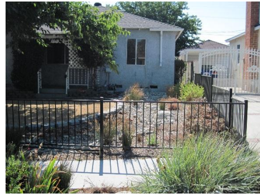
Residential LID retrofit in the form of a xeriscaped infiltration swale
