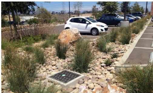
Recently constructed biofiltration in a parking lot
