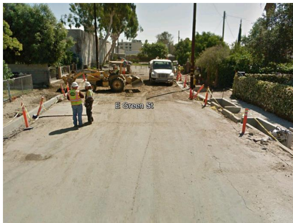
Green Street infiltration basin under construction (Source: Google Earth)
