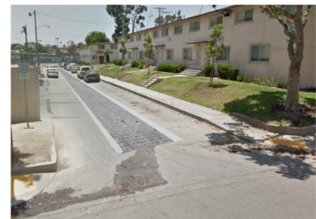
Rendering of a proposed bioswale at a local playground (top) and rendering of a proposed permeable alley (bottom)
