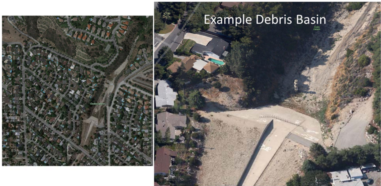
Figure A-1. Example debris basin. There are 162 such structures at the base of mountain canyons at the natural-urban interface. The overflow weirs are the start of the storm drain network.
