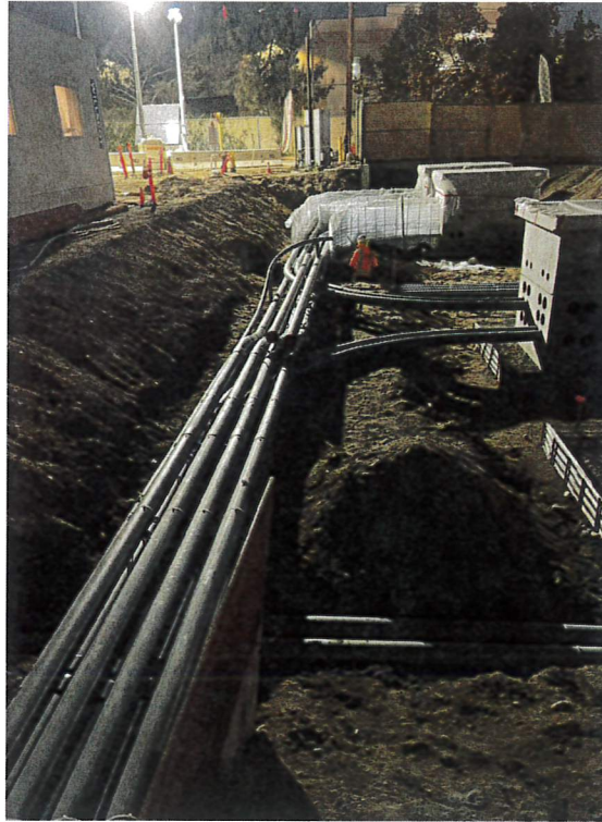
Conduit installation at Airport switchyard
