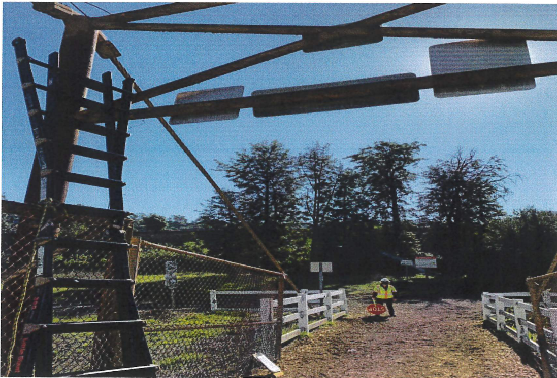
Photo 6_Ladder Used for Weld Inspections
