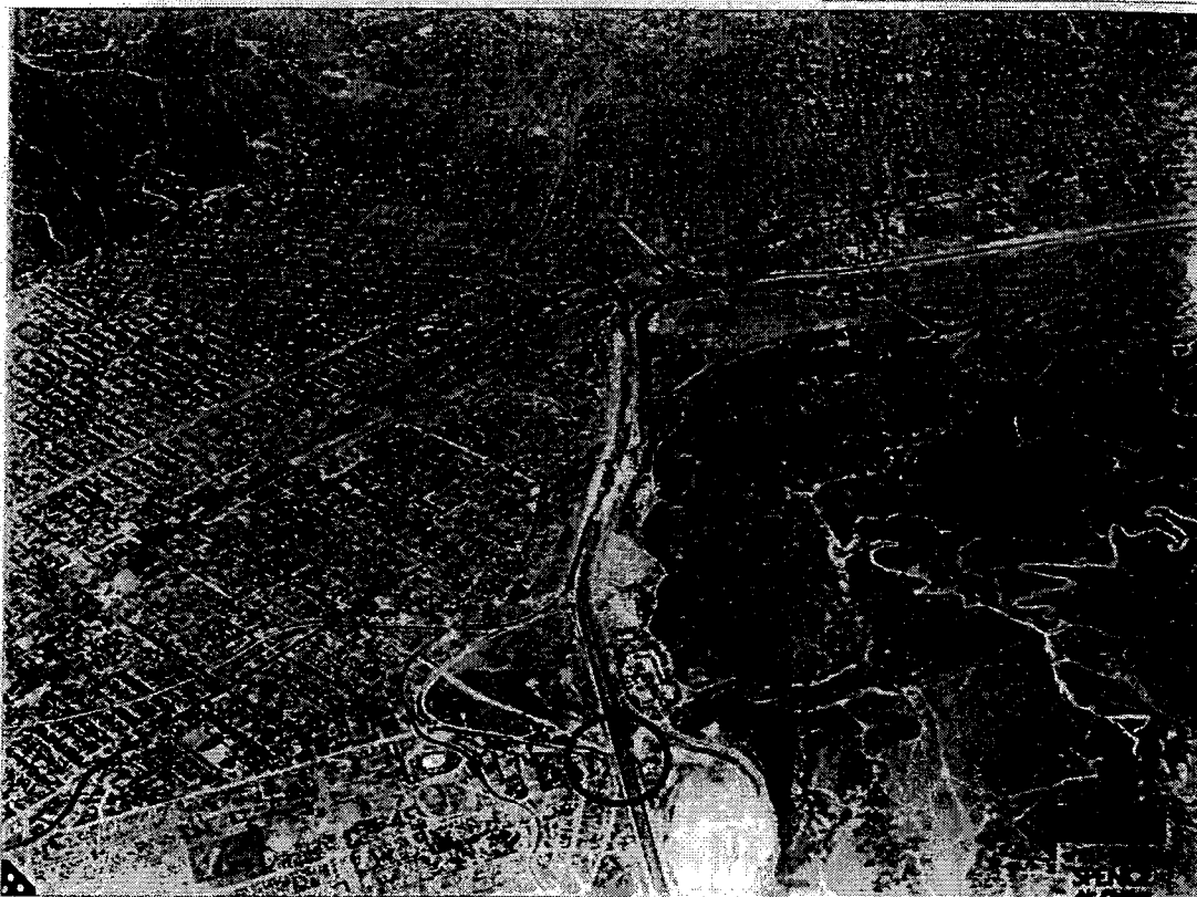
Figure D: Historic aerial photo, Mariposa Street Bridge circled red (University of California Los Angeles Air Photo Archives, 1946)
