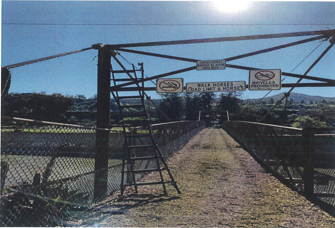
Photo 5_Ladder Used for Cable Inspections
