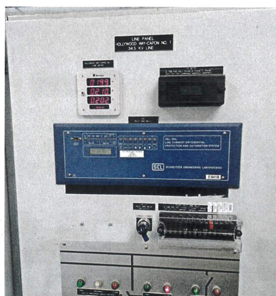
After Installation (New Relay)
