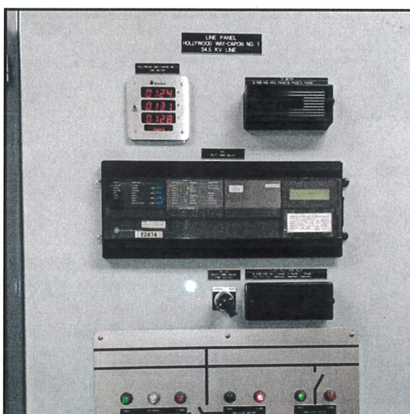
Before Installation (Old Relay)
