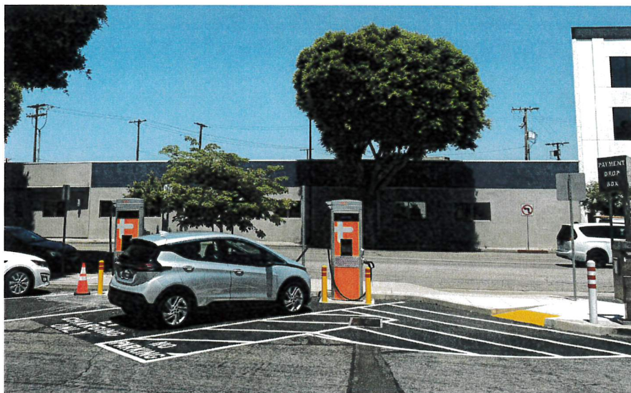
Two new DC fast chargers are now publicly available in the Magnolia Blvd. customer parking lot.
