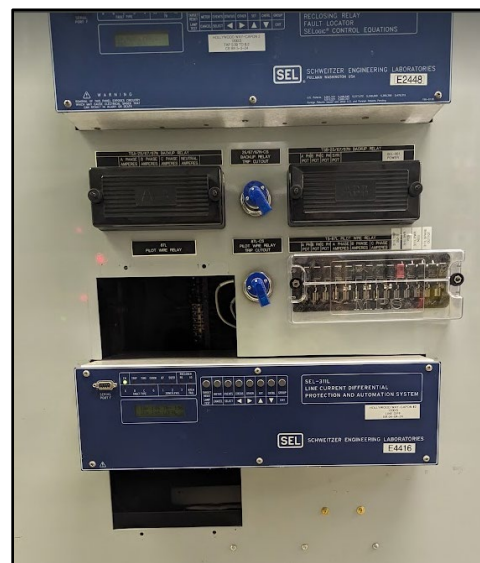
After Installation (New Relay)
