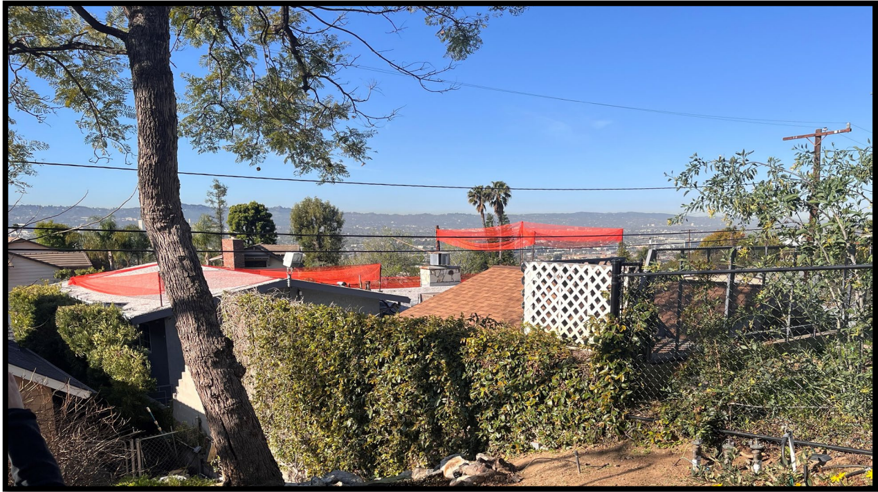
Figure 9: View of the existing residence from neighboring property 1012 N. Sunset Canyon Dr., looking towards the story poles where the second-story additions will be constructed.
