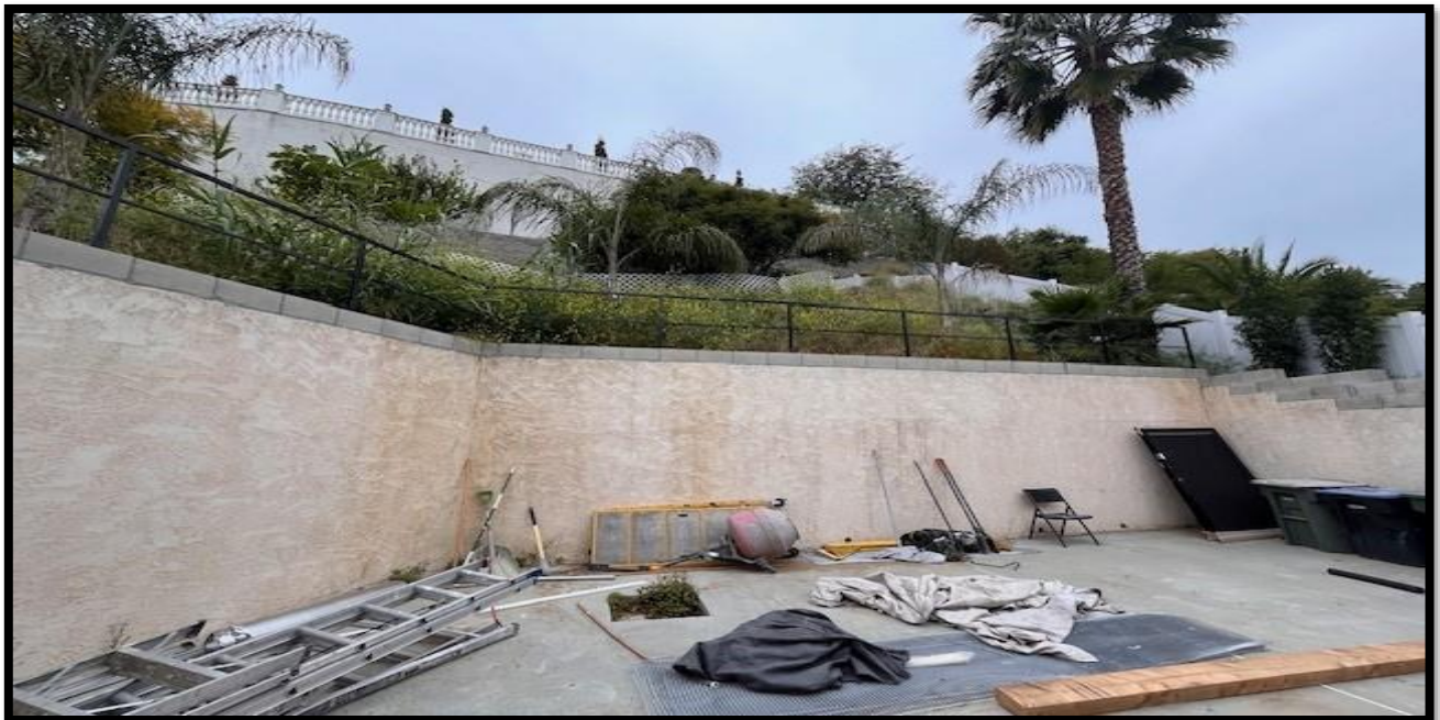
Figure 12: View of property 1038 Sherlock Drive from the rear yard of the project property.
