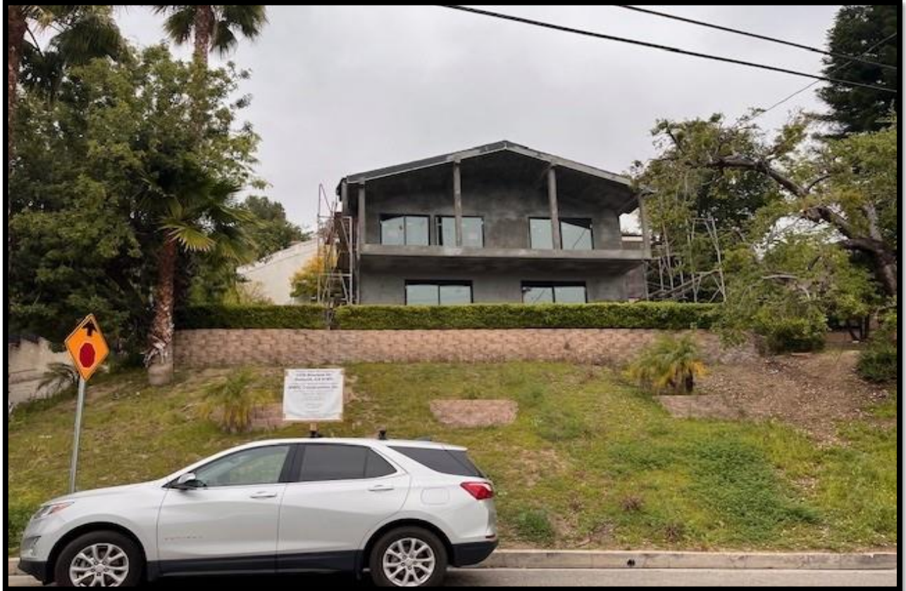
Figure 6: View of the front property looking north where the proposed stairs and front deck will be constructed.
