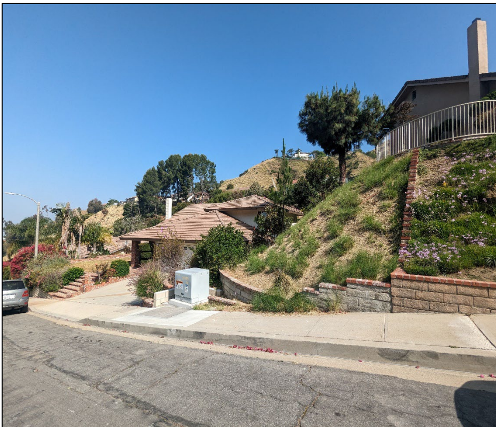
East view of story pole installation, from Brace Canyon Road (front).
