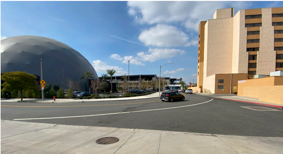
View of the dome south of the Project Site from the eastern side of Avon Drive looking west toward Hollywood Way with the southern portion of the Project Site shown on the right-hand side of the photo
