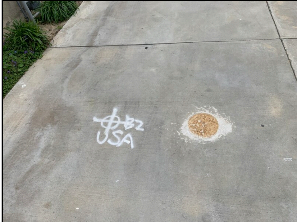
Photo 26: View of USA ground marking located on the concrete access way between 2325 and 2331 N. Fairview St.
