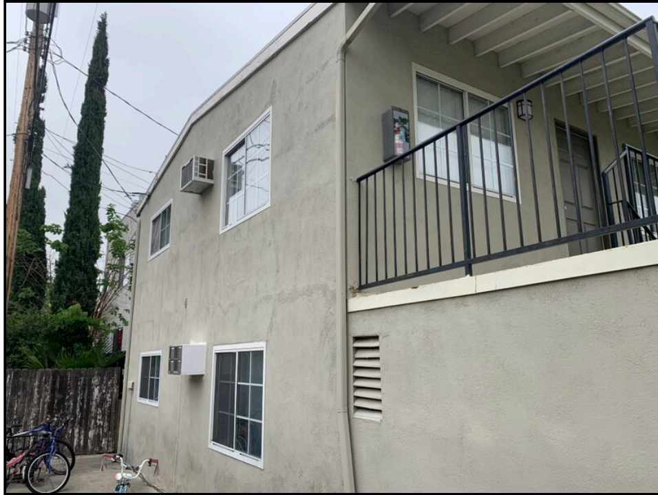
Photo 1: View of the west portion of multi-tenant residential structure.
