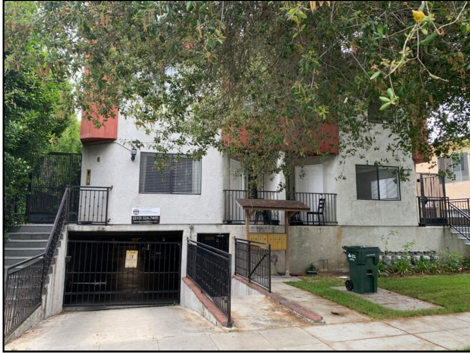
Photo 27: View of the north adjoining residential structure looking to the west.
