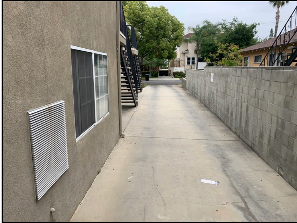
Photo 21: View of concrete paved access way located south of 2321 North Fairview Street looking to the east.
