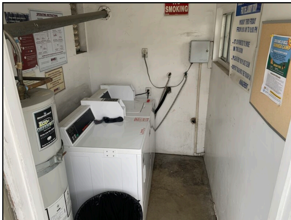
Photo 5: View of laundry room onsite at 2335 North Fairview Street.
