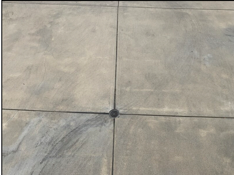
Photo 4: View of storm drain located in the concrete paved parking area.
