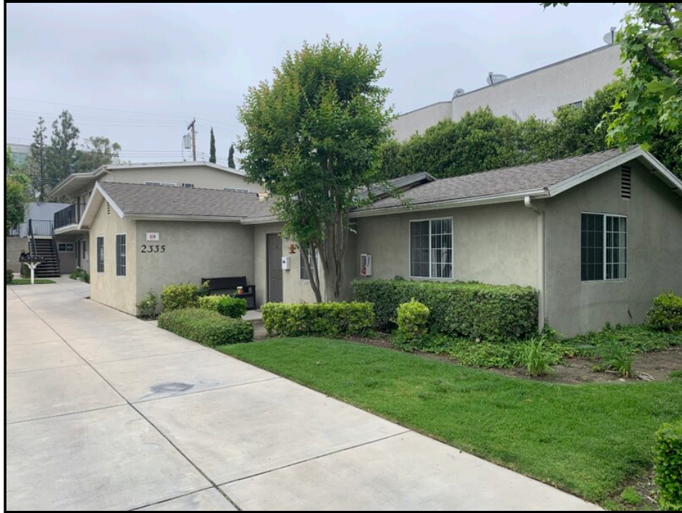
Photo 3: View of single family residential structure (2335 N. Fairview St.)
