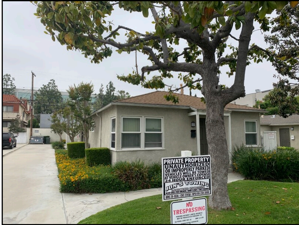
Photo 10: View of single-family residential structure 2331 North Fairview Street looking to the northwest.
