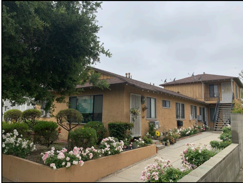
Photo 29: View of the south adjoining residential structure looking to the west.
