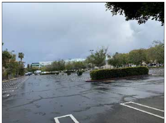
30. Parking lot in northeast corner of subject property
