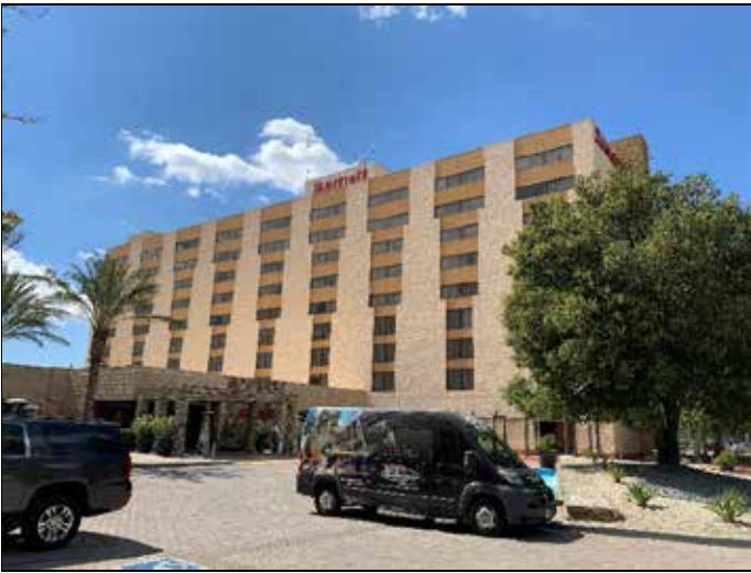
1. West Tower guestrooms
