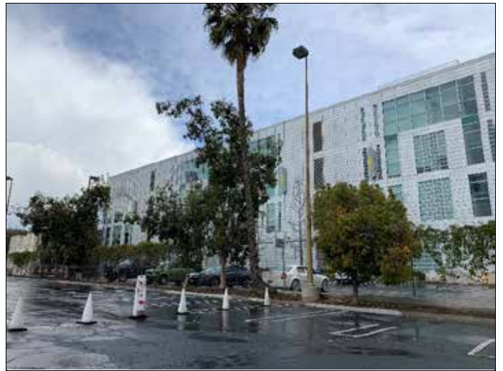
34. Adjacent property to east – 3100 Thornton Avenue
