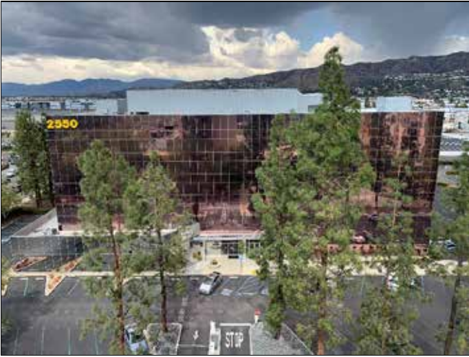
31. Adjacent property to north – 2550 North Hollywood Way
