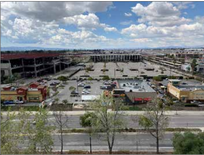
33. Adjacent properties to west
