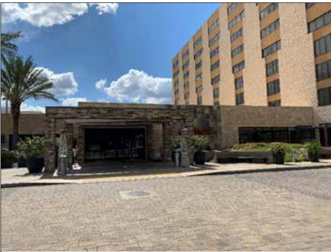
3. Entrance to main lobby on west side of building
