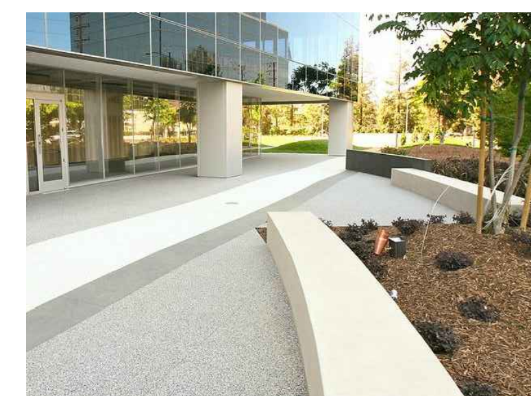
7 CAST-IN-PLACE CONCRETE SEATWALLS W/ LITHOCRETE FINISH
