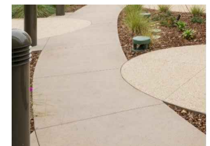
6 CAST-IN-PLACE CONCRETE SIDEWALK W/ TOPCAST FINISH
