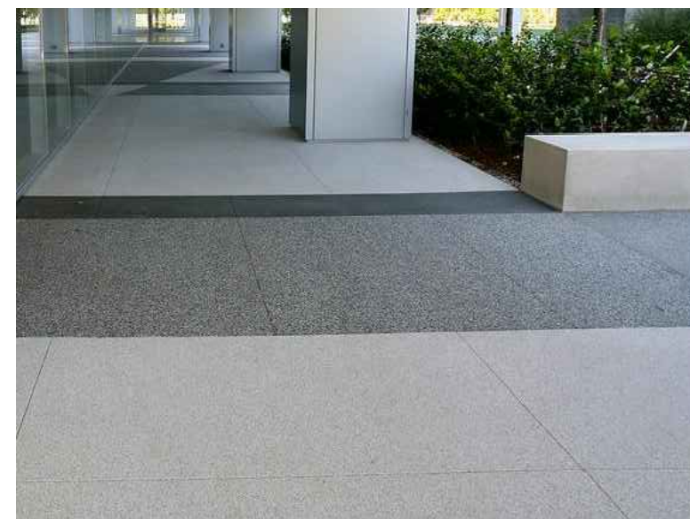
1 CAST-IN-PLACE CONCRETE W/ LITHOCRETE FINISH
