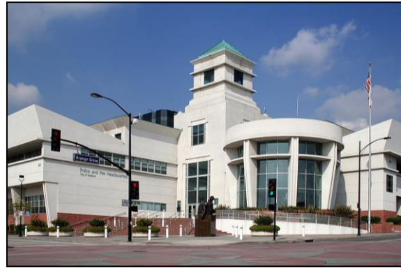
The headquarters building for both the Burbank Police and Fire Departments is located at the intersection of North Third Street and Orange Grove Avenue.
