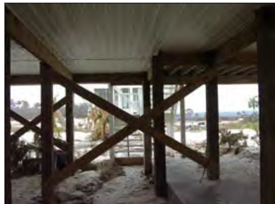
Figure 2. An open foundation.
