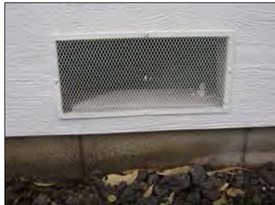
Figure 1. A closed foundation with a cripple wall (FEMA field team).
