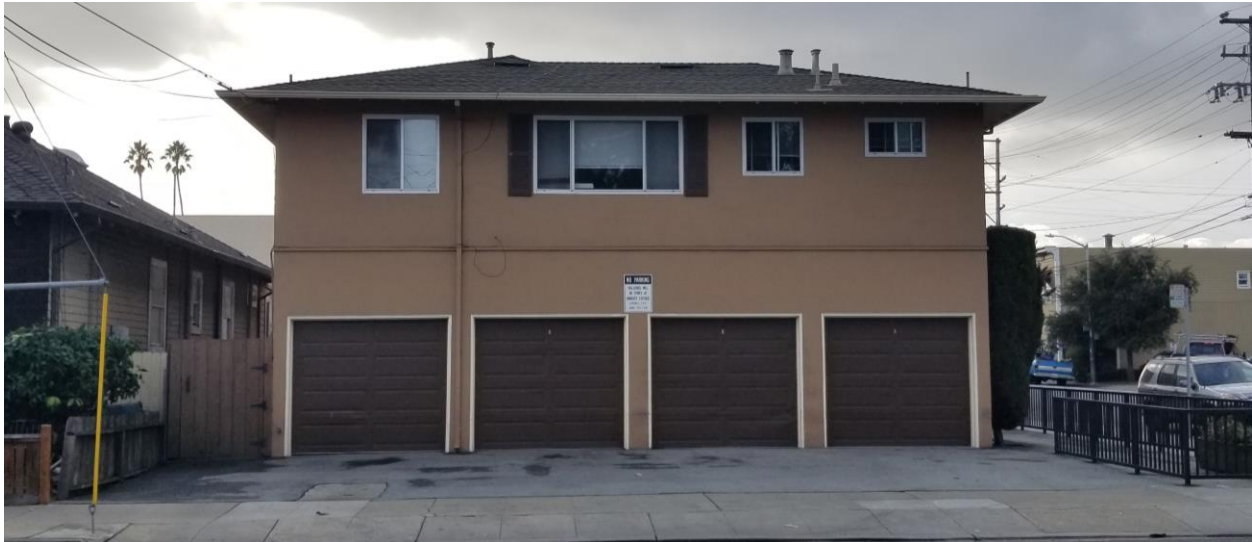
Figure 5-6 Example of the short-side-open building with parking areas on a short side of the building. The parking area shown is enclosed by garage doors.
