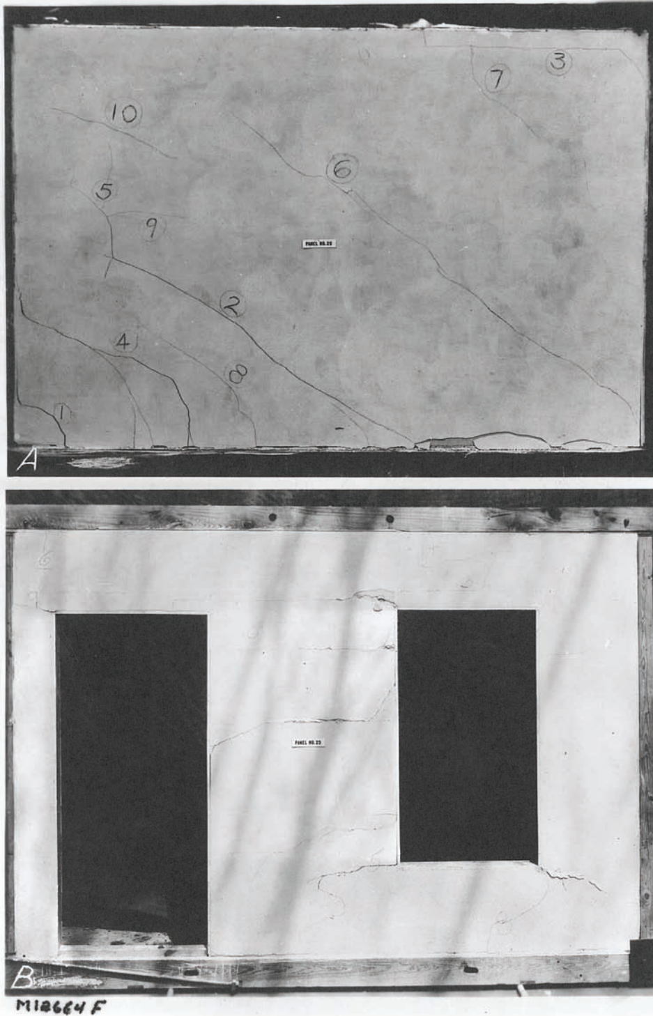
Figure D-31 Photos of characteristic cracking at completion of Forest Products Lab testing (from Trayer, 1956).
