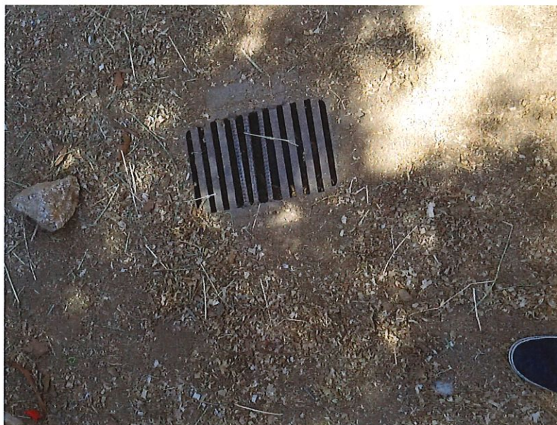
Drainage inside the property.
