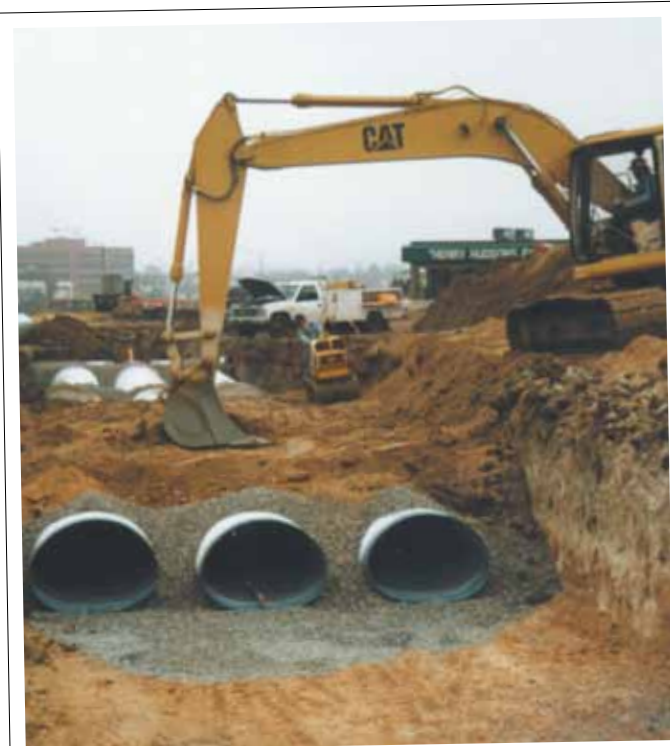
Pipe-arch for low profile application.
