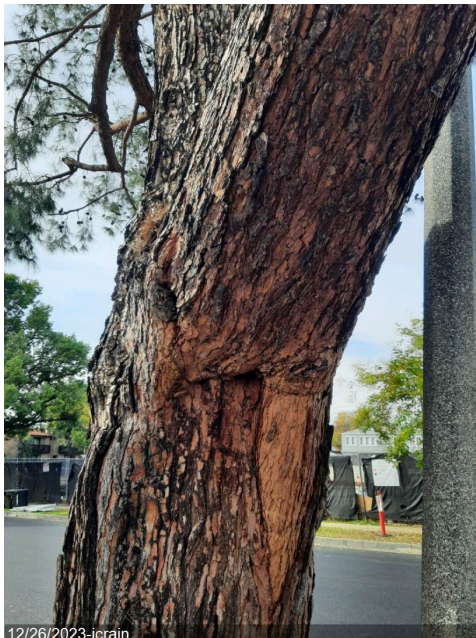
Cavity beneath the attachment of main scaffold.
