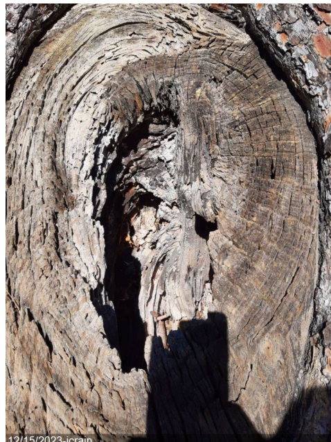
Decay in the same cavity
