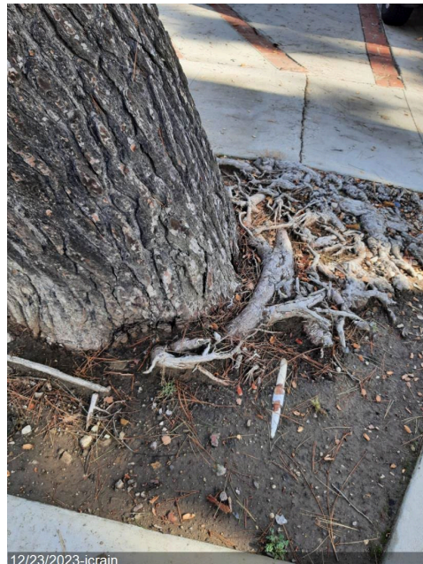
Visible circling roots.
