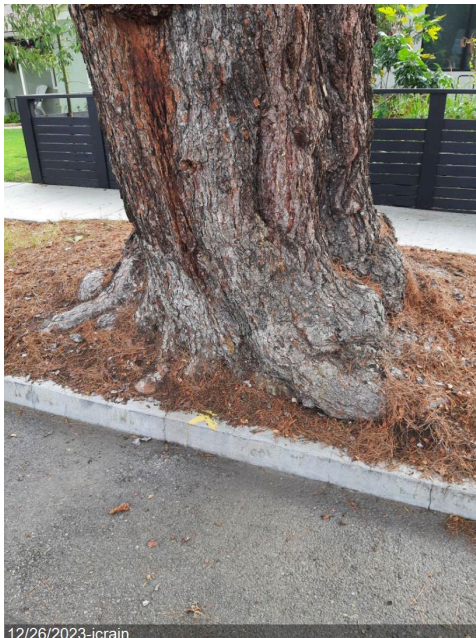
Signs of decay in visible roots.
